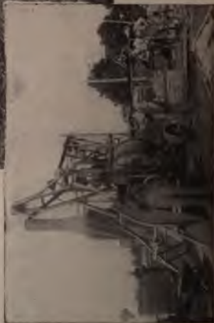
The road here illustrated as under construction is known as the Pacific highway, and is located in Lewis county, Wash. It is being laid in two courses, the base being of a 1:3:6 mixture with egg gravel, 5 inches thick at the center and 3½ inches at the sides. The surface is a 1:1:2 mixture with pea gravel. The width is 16 feet. A Koehring street paving mixer is being used.
